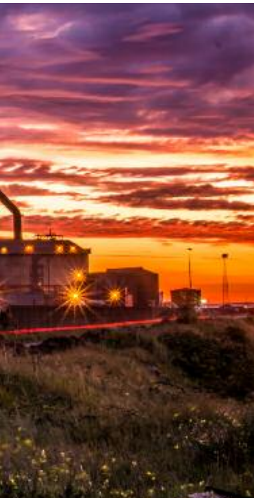
Once cooled, a furnace cannot be brought back.
