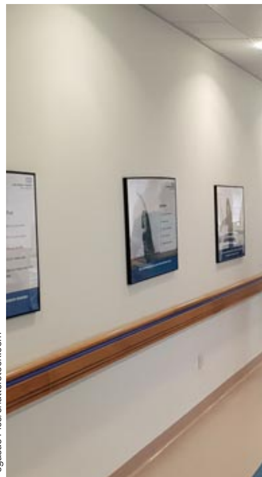
Great Western Hospital, Swindon.
